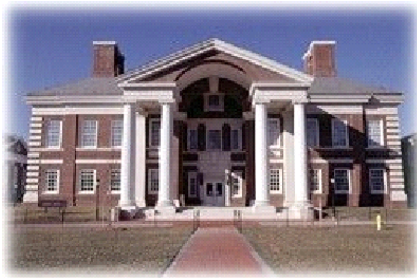
Figure 7.1: Can we make use of prior models of specific building elements to estimate structure?
